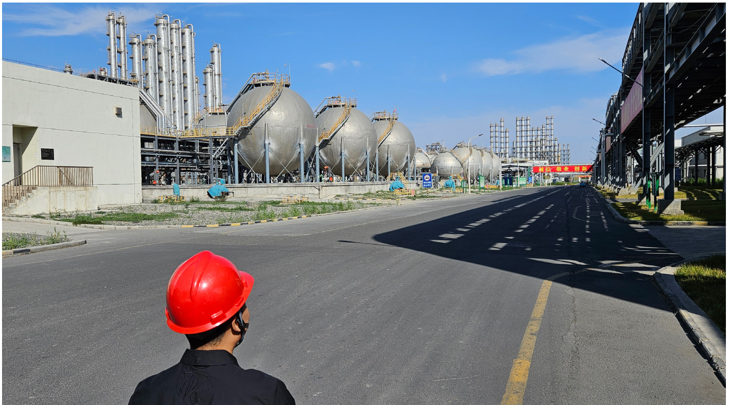
Xinjiang province, China. Site tours of Daqo New Energy's factories in the region. The large spherical tanks contain hydrochloric acid, while the cylindrical towers are used for distillation, both needed for the production of polysilicon which is the most important material used in solar modules.
